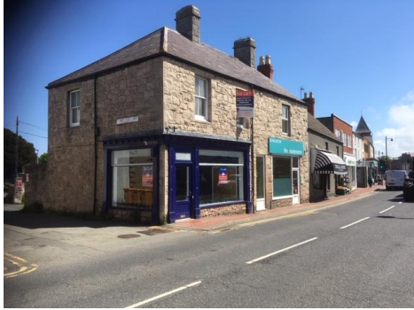
38 Market Street ABERGELE
